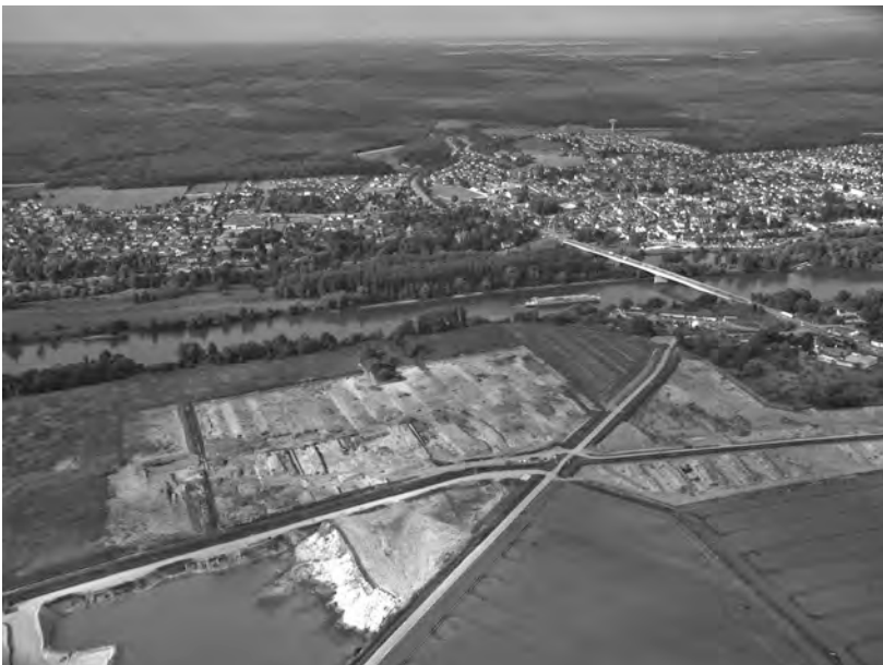
FIGURE 1: AERIAL VIEW OF THE EXCAVATION (H. PAITIER).
